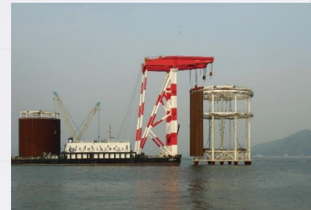
Offshore Heavy Industry and Port Machinery Manufacturer and Service Provider
